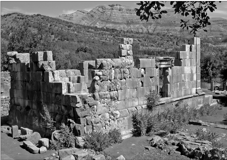
Fig. 8 The Hellenistic and Roman sanctuary at Yanouh, today used as a monastery of Mar Girios: a a recent photograph showing the remains of the large Roman temple. – b a plan showing the two large courtyards, and the buildings from Hellenistic to Byzantine times. – c a reconstruction of the Roman podium temple in the courtyard with the porticus. – (a. c after Aliquot 2009, figs 137. 135; b after Charpentier 2020, fig. 22, see also fig. 20 for a section).
